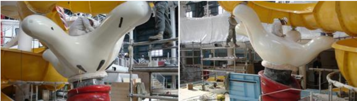
FormaShape attaching the slide flume to the supporting hand
