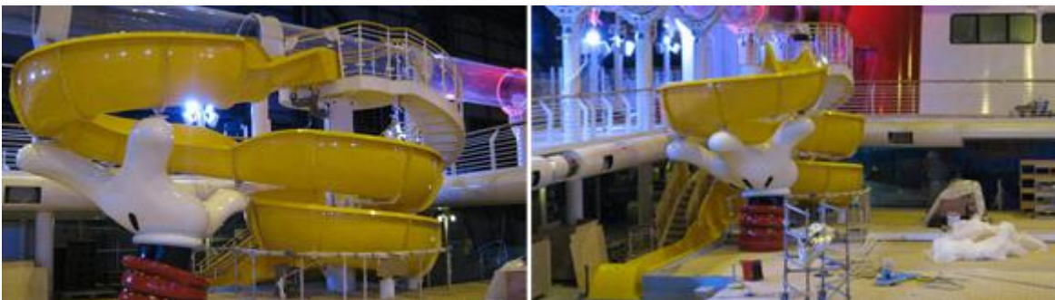
The completed slide just before it debuted on its maiden voyage in April 2011
